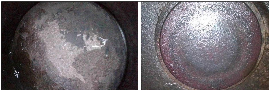
Figure 10: Borescope photographs examples of overall condition of all six piston/cylinder assemblies.
