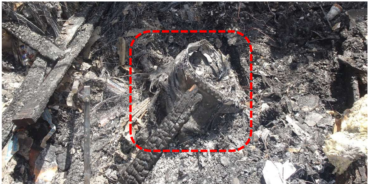
Figure 9. The tail boom connection to the main fuselage as seen in the building.
