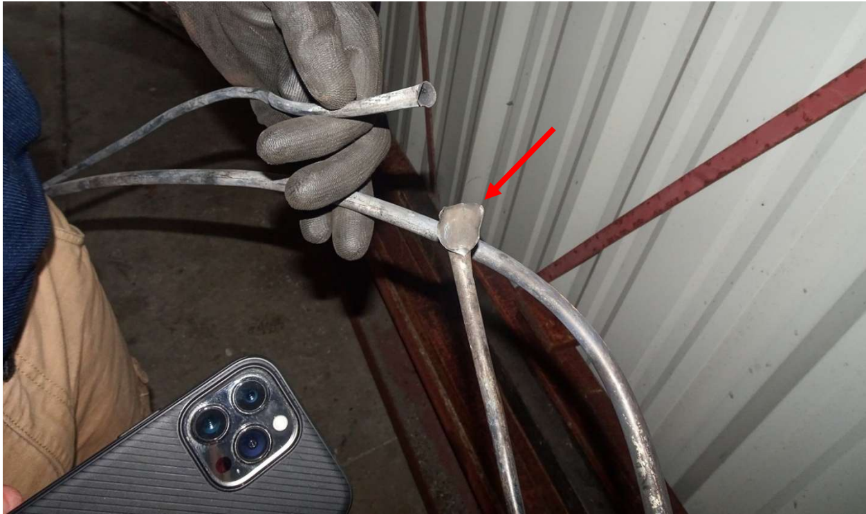
Figure 14. The tail rotor hydraulic actuator pressure line that exhibited a burst-like appearance.
