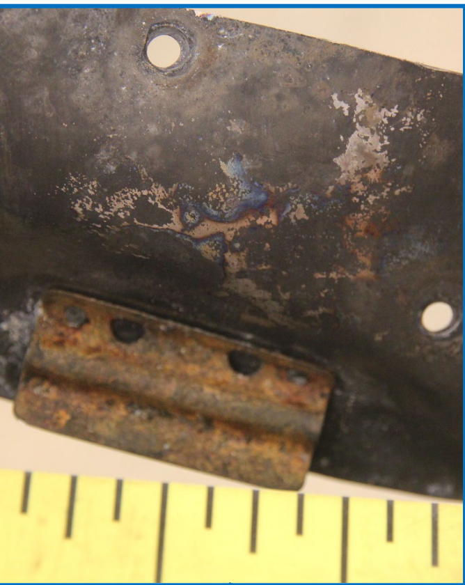
#1 Engine Intake Firewall, Inboard
