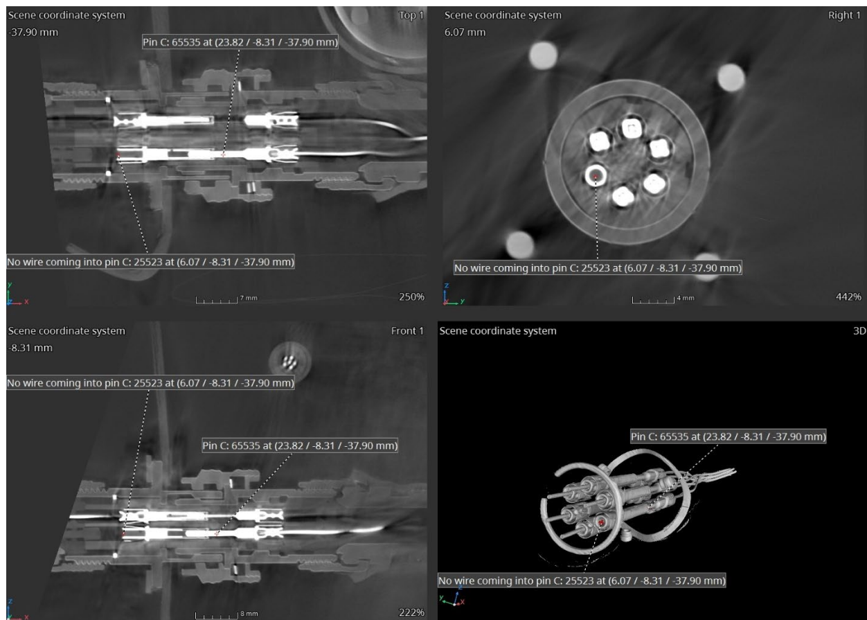
Figure 15. Fuel shut-off valve – electrical connector – pin C. (225 kV)
