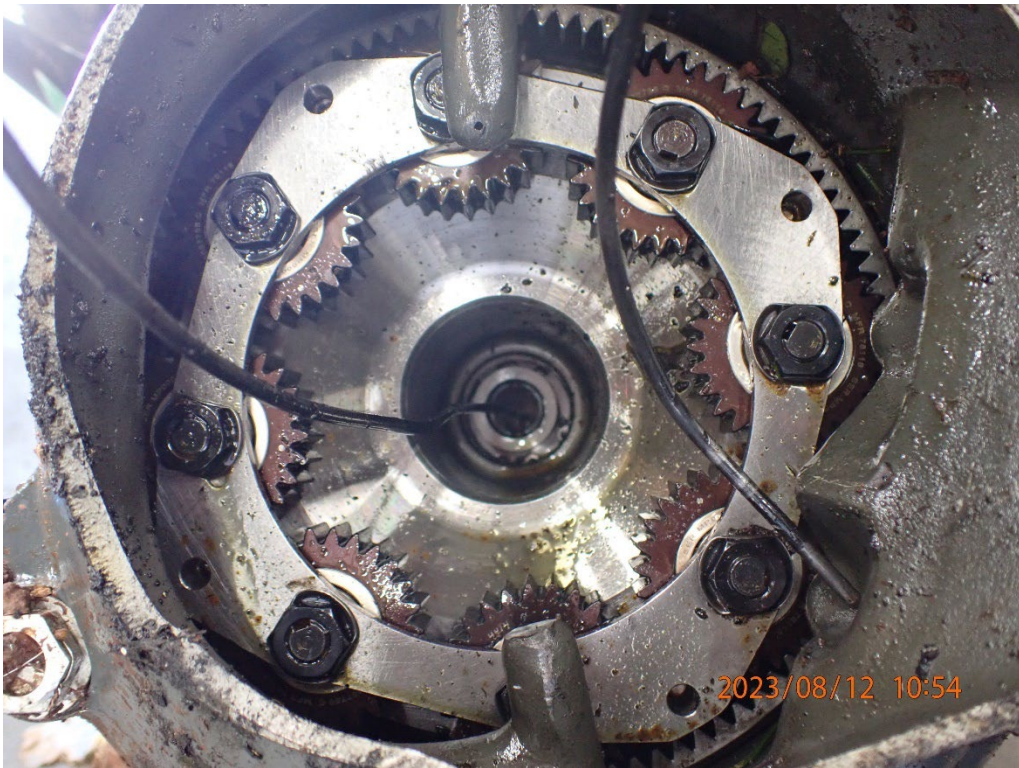
Photo 42: View of the gears inside the propeller gearbox.
