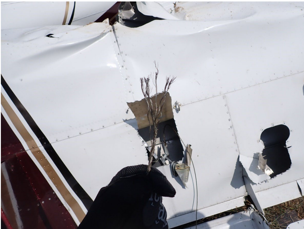
Photo 10: Aileron through cable end that was attached to the left aileron bell crank.
