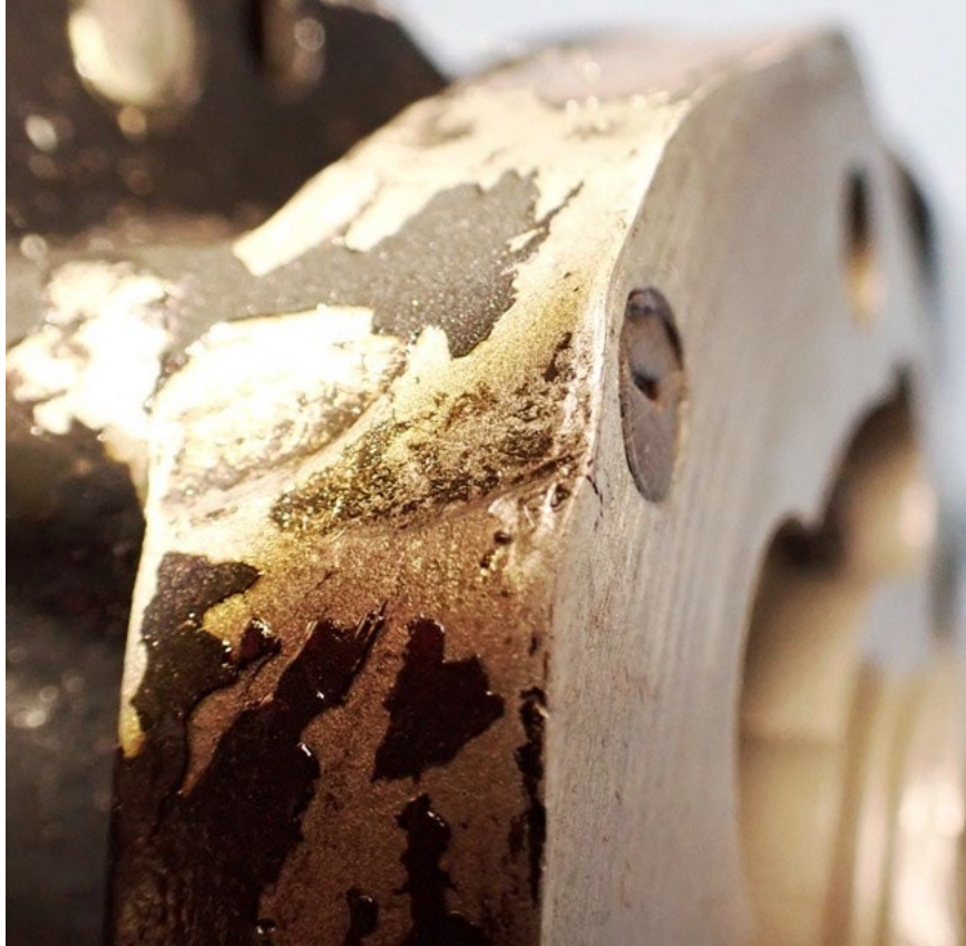
Photo 7: Governor mounting flange impact damage on edge. (Hartzell Photo)
