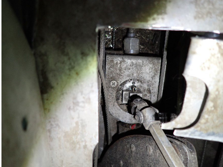
Figure 13 View of the Interior Skin Beneath the Fuel Selector Valve
