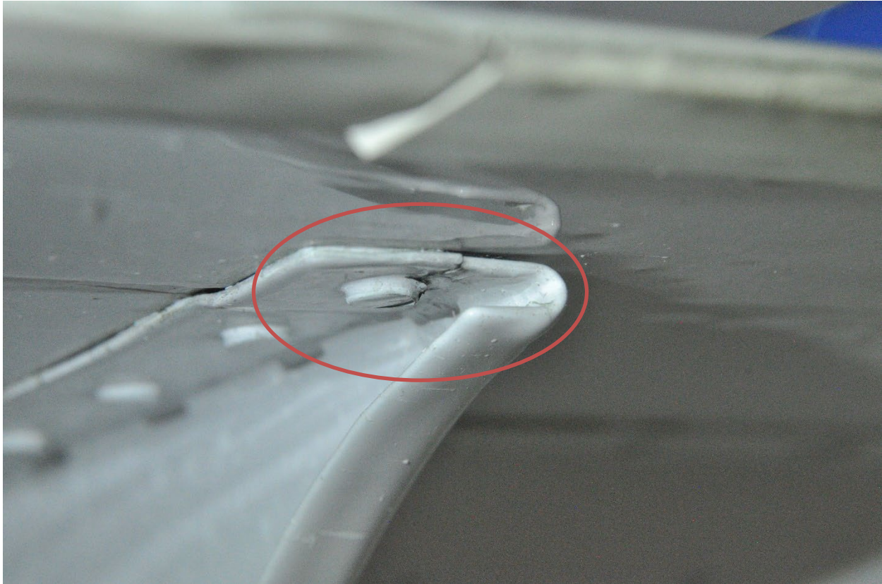
Figure 9. Example of flap cove rib cracking near aft rivet (crack is circled in red)(picture location near Right Wing Station 106)(courtesy of Tamarack Aerospace Group).
