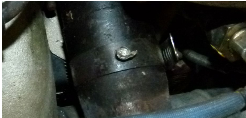
Figure 27 No. 4 Exhaust Gas Temperature Probe Mount Location with Installed Clamp and Remainder of Fractured probe
