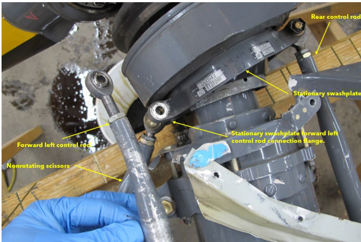
Figure 5. Photo of the upper controls showing the disconnected forward left control rod from the stationary swashplate.
