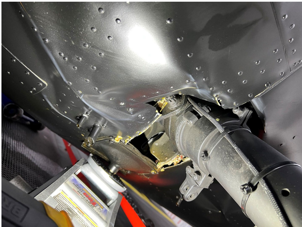
Right Rear Aft Cross Tube damage
