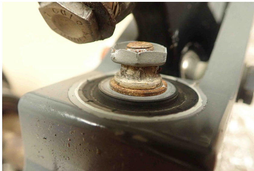
Figure 2 – Corrosion to hardware
