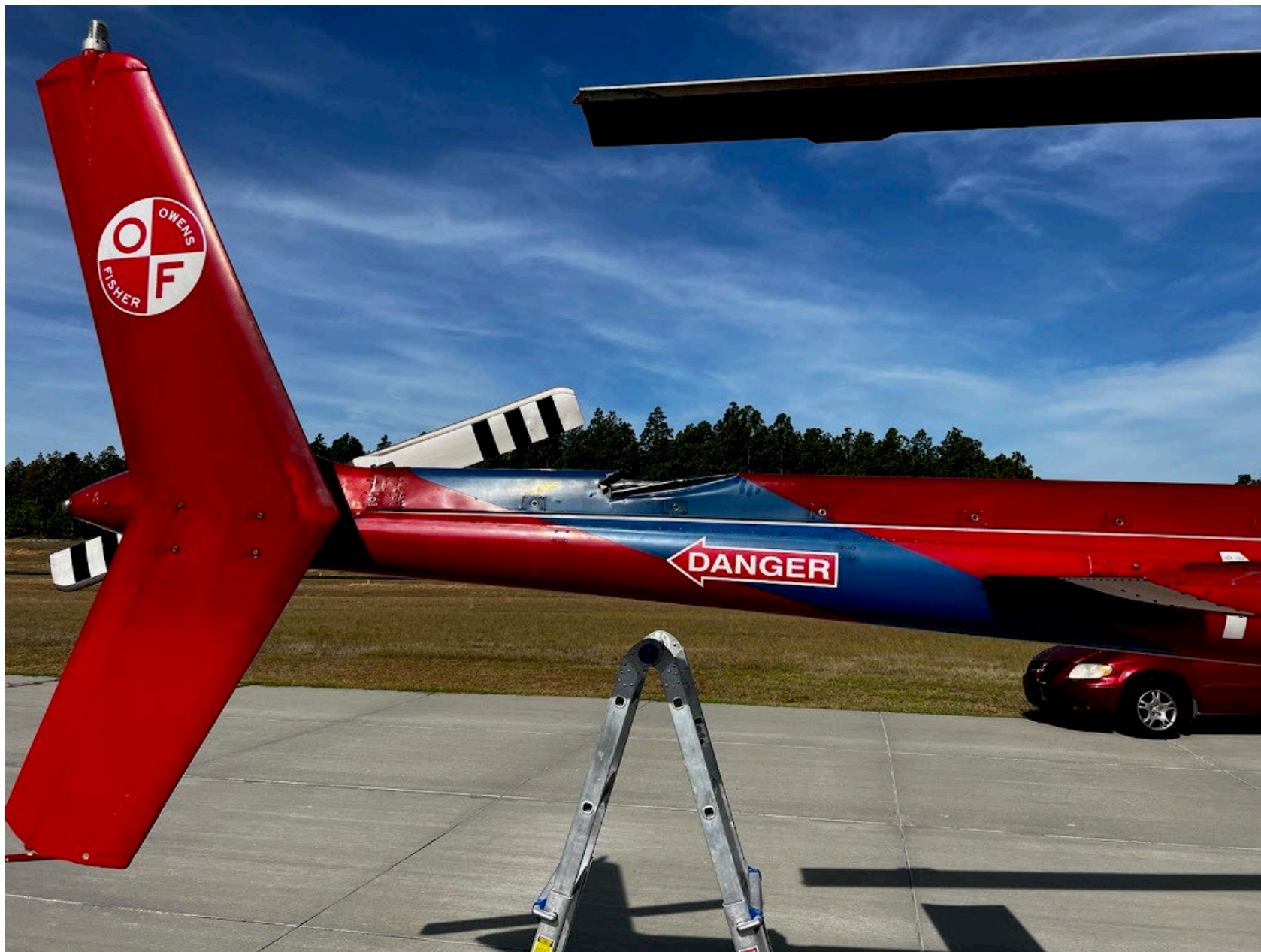
Photo 1 – Right Side View of Damage to Tail Boom (FAA)
