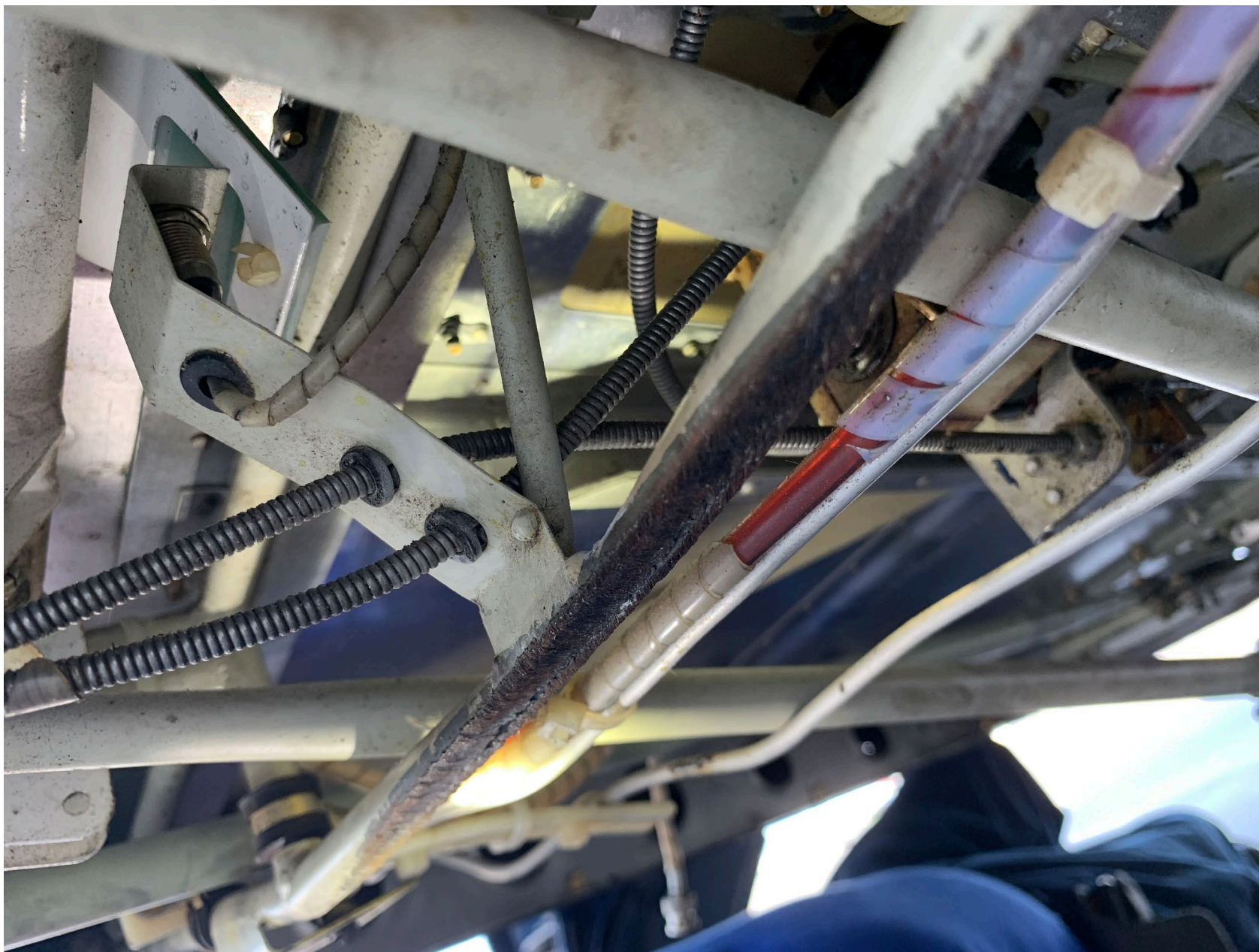
Photo 5 – FAA Digital Photograph. View Depicting the Damage to a Tubular Steel Truss Primary Structure Which Required Major Repair and Classification as an Accident.
