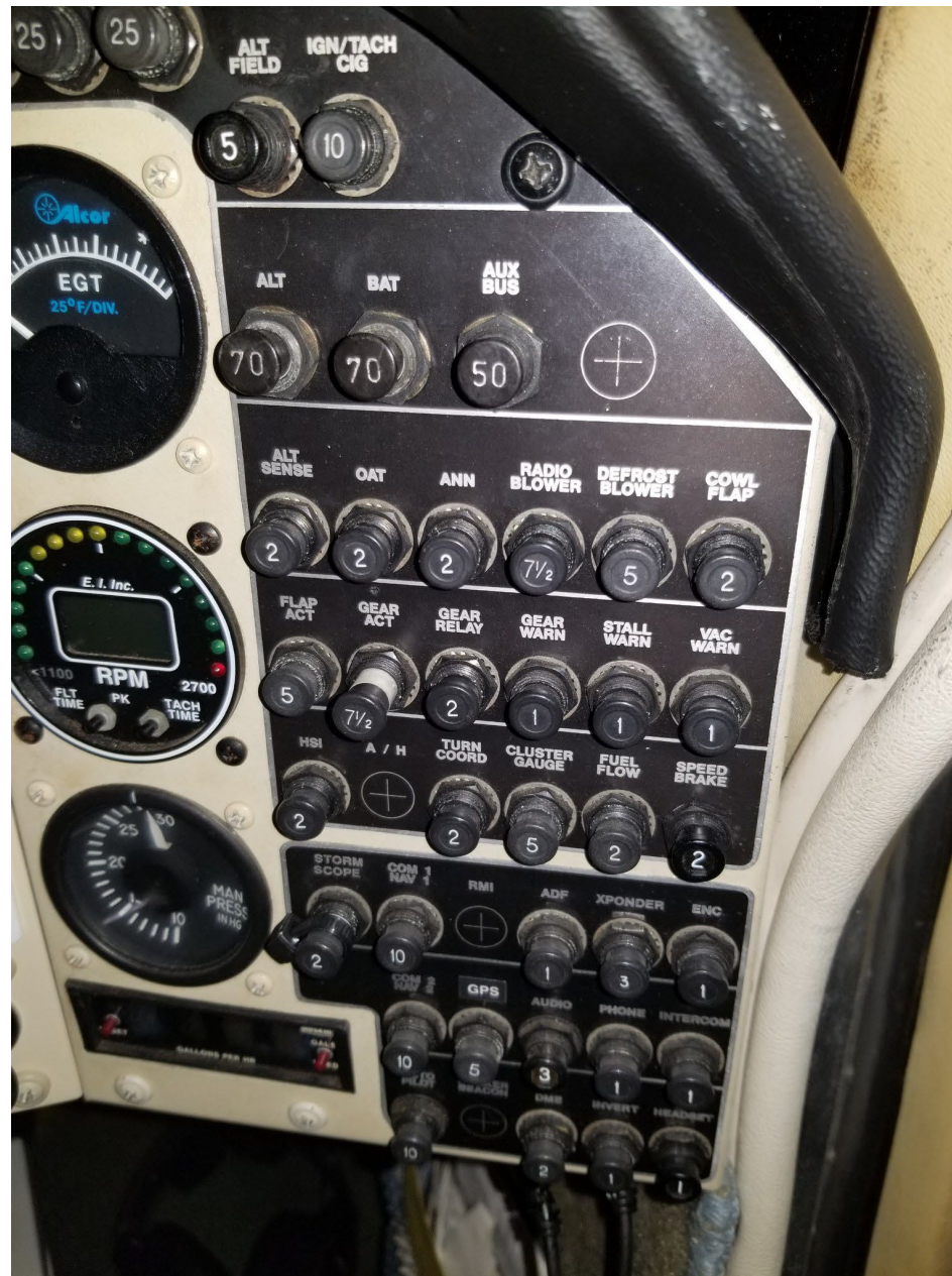
Photo 2 - Digital Photograph From Charleston Air Force Base Airport Operations. View of the Circuit Breaker Panel Showing the Gear Actuator Circuit Breaker Tripped.
