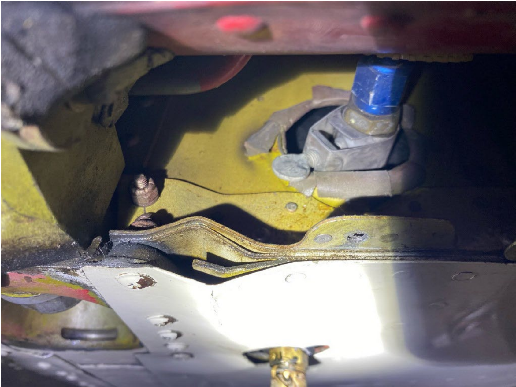
Photo 2 – Wrinkling of Lower LH Wing Structure
