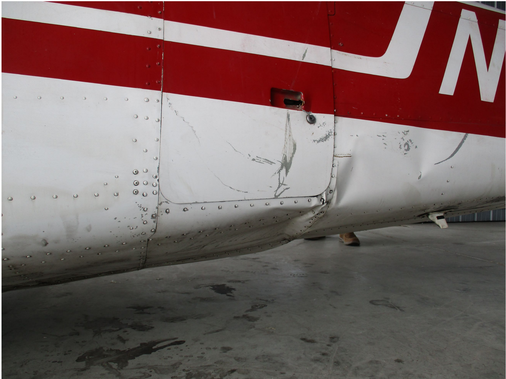
Photo 4 - FAA Digital Photograph. Left Side View of the Left Side of the Fuselage. Note the Compression Buckling adjacent to Door and Lower Portion of the Fuselage.
