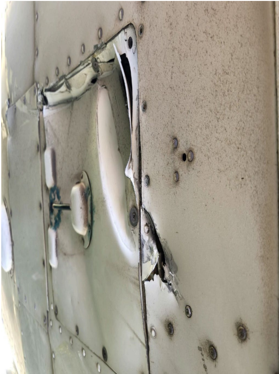
Photo 2: Damage to the airplane's fuselage (Photo Courtesy of FAA)
