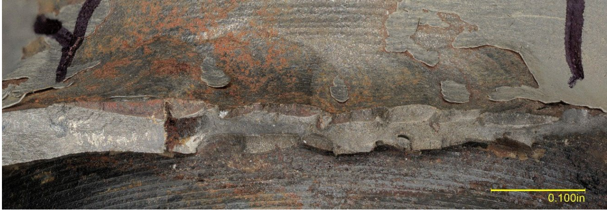
Figure 7. Closer view of the thumbnail cracks on the torque tube fracture location circled in Figure 6.
