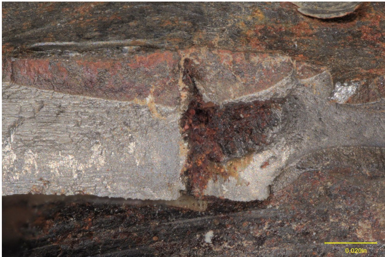
Figure 9. View of the largest thumbnail crack from the left side of Figure 7.
