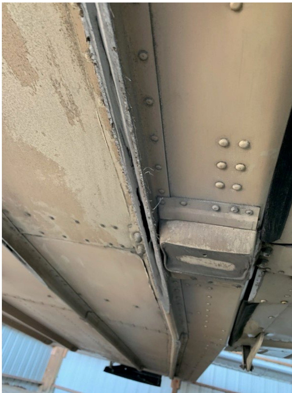
Photo 2 – external longerons (owner)
