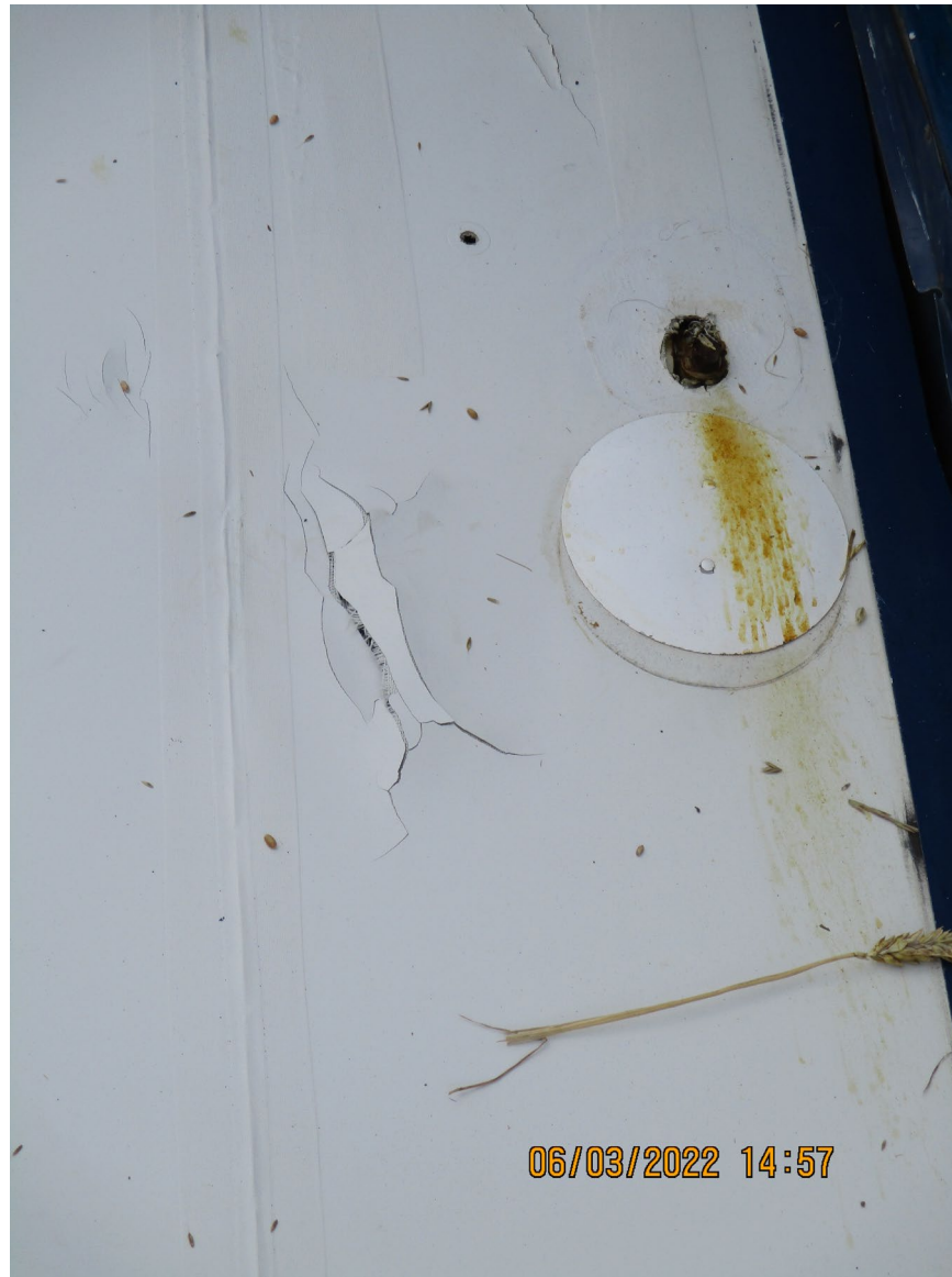
Photograph 3 - View of staining aft of right wing fuel sump. (Courtesy of FAA)
