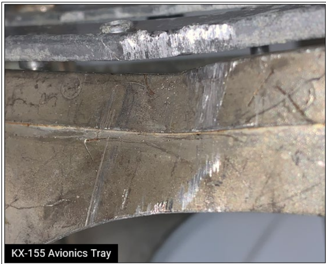
Figure 6: View of the KX-155 avionics tray and its bottom side. This side was the nearest surface to the elevator bell crank. Significant scrapping, metal polishing, and deformation of the tray was observed.
