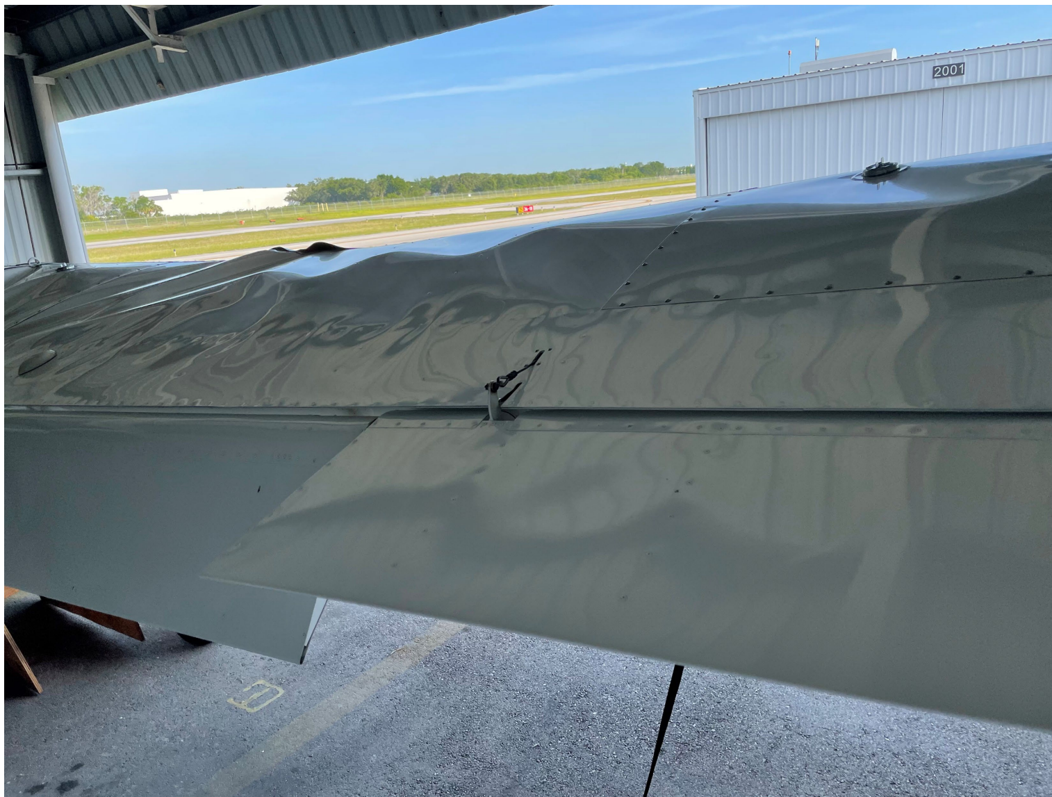
Photo 5: Overview of the right wing damage, trailing edge (FAA Photo)
