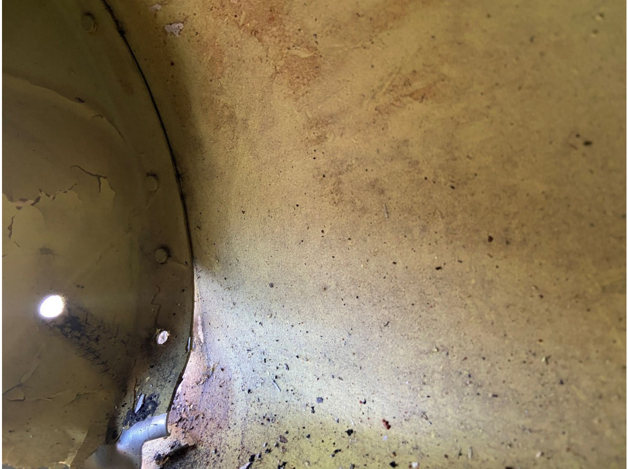
Photograph 3 – Interior view of tail section damage.
