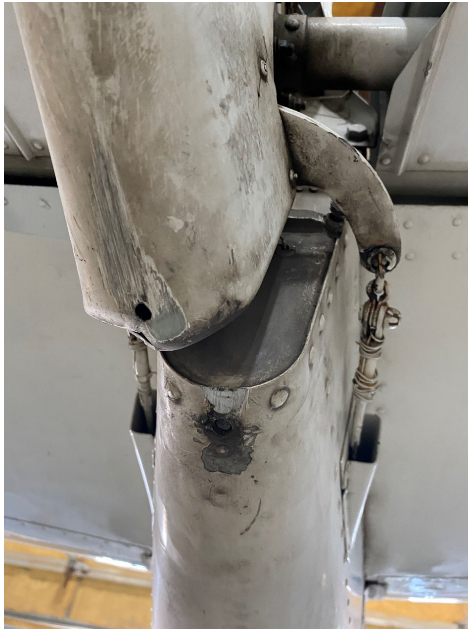
Photo 4: View of the rudder control surface damage (Photo Courtesy of FAA)
