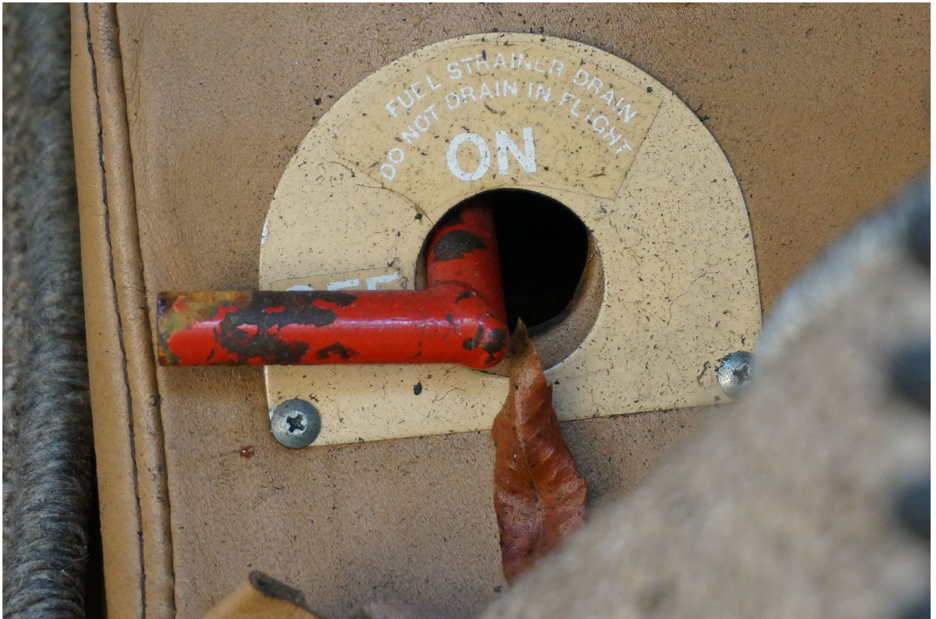
Photo 11 – Fuel Strainer Drain
