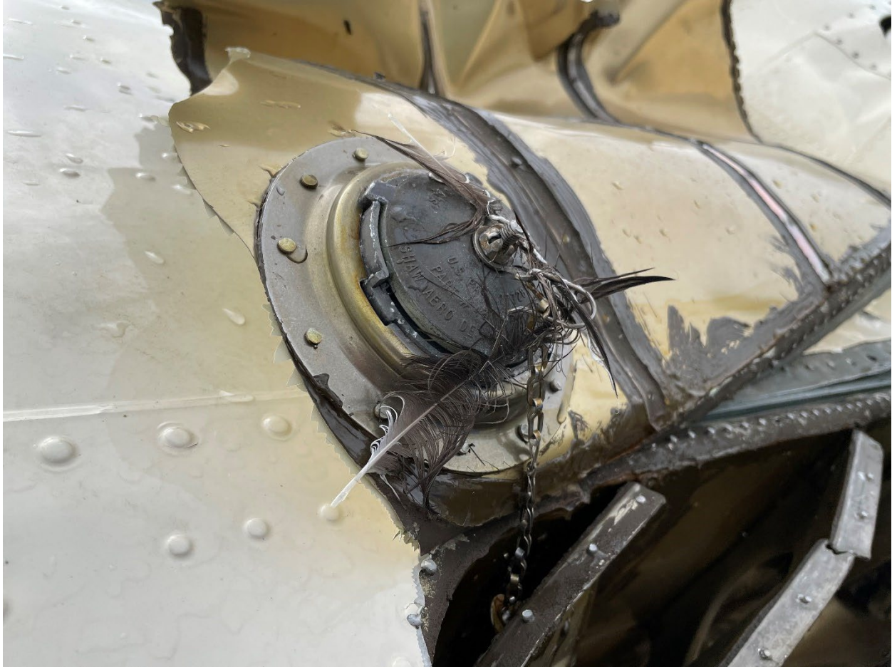
Figure 1 - Right Wing Tank Fuel Cap / Feather Remnants
