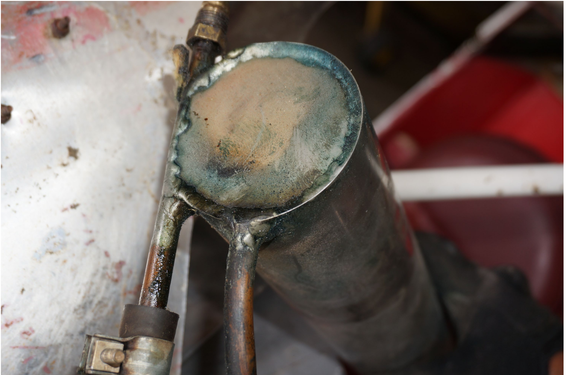
Photo 16 -Bottom of Header Tank
