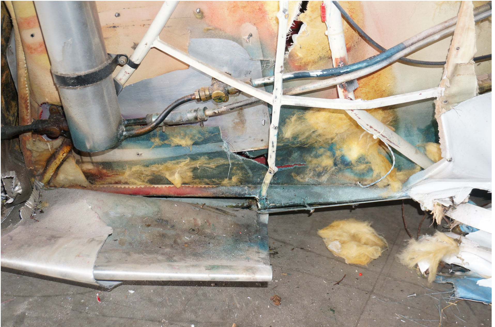
Photo 15 – Close Up of Modifications to Header Tank
