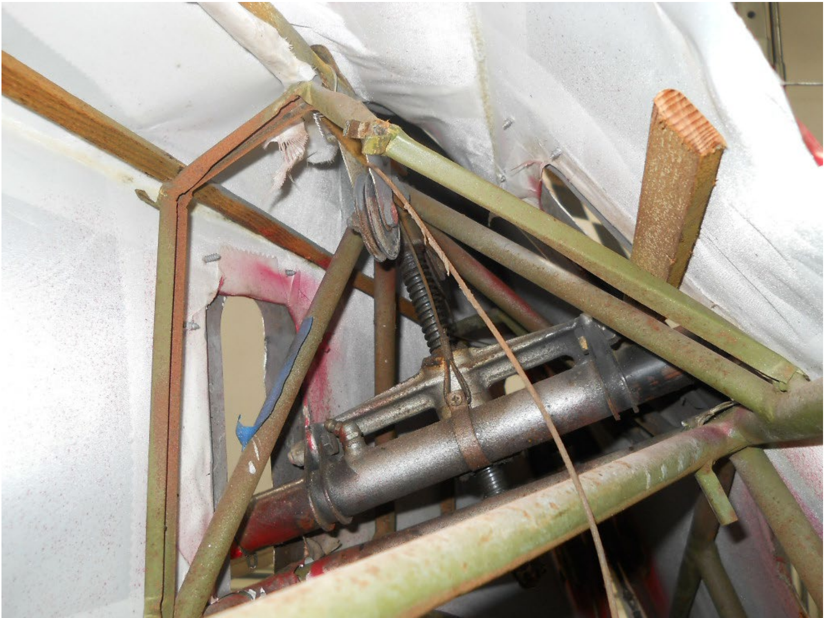
Photo 3 – Horizontal Stabilizer Trim Jackscrew
