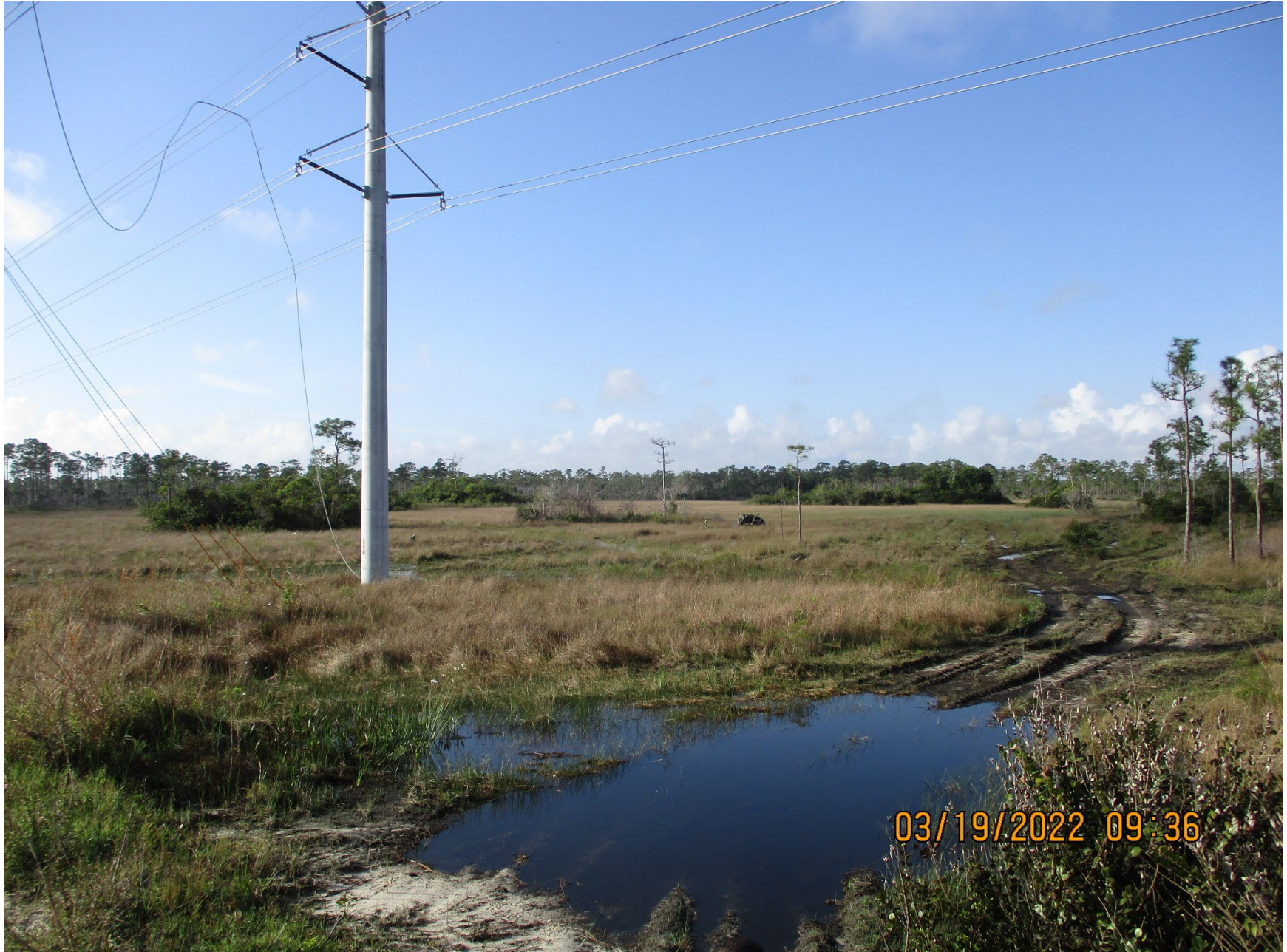
Photo 1 – cut powerlines with main wreckage in background
