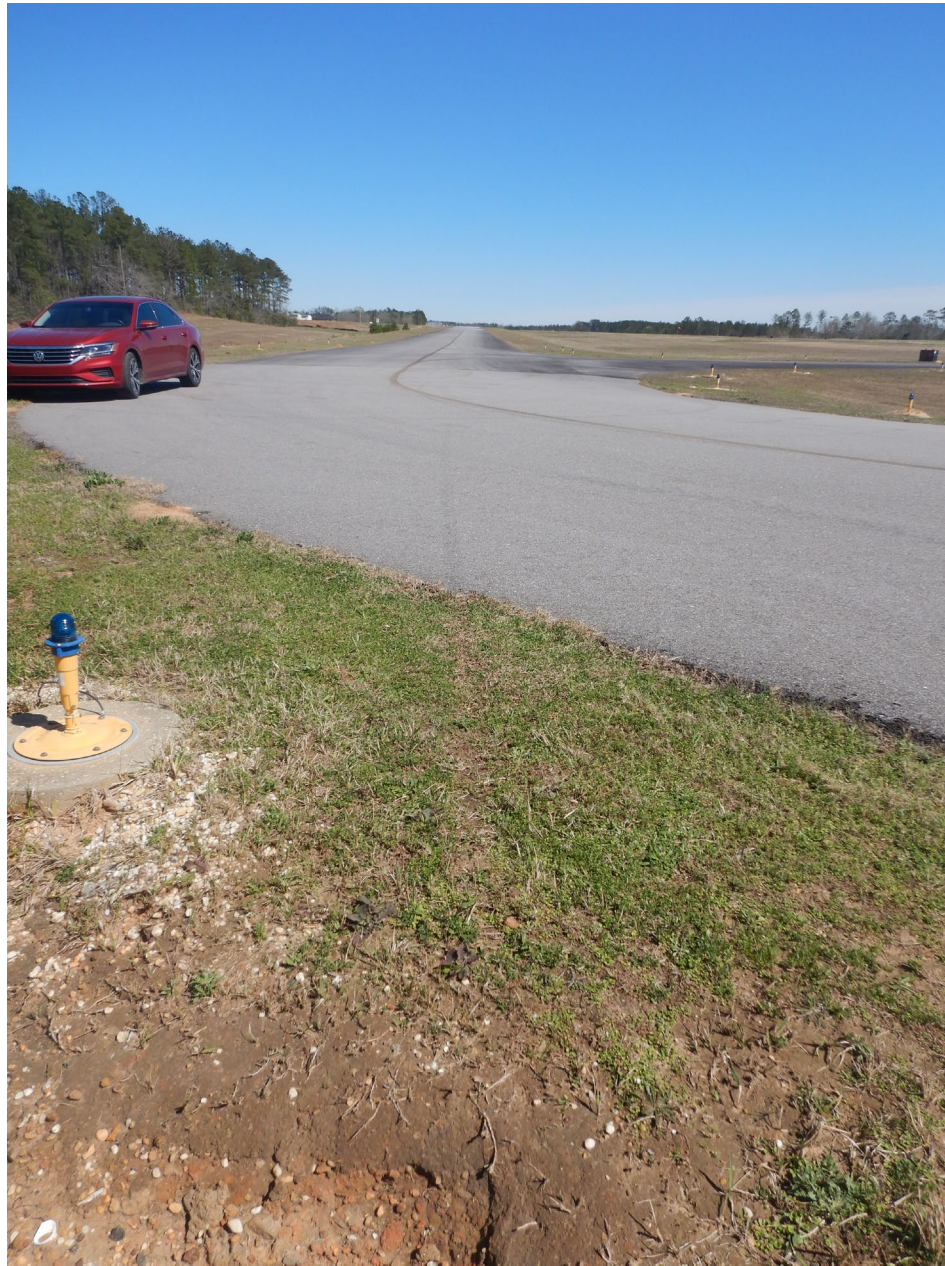
Photo 2 – Continuation of Skid Marks
