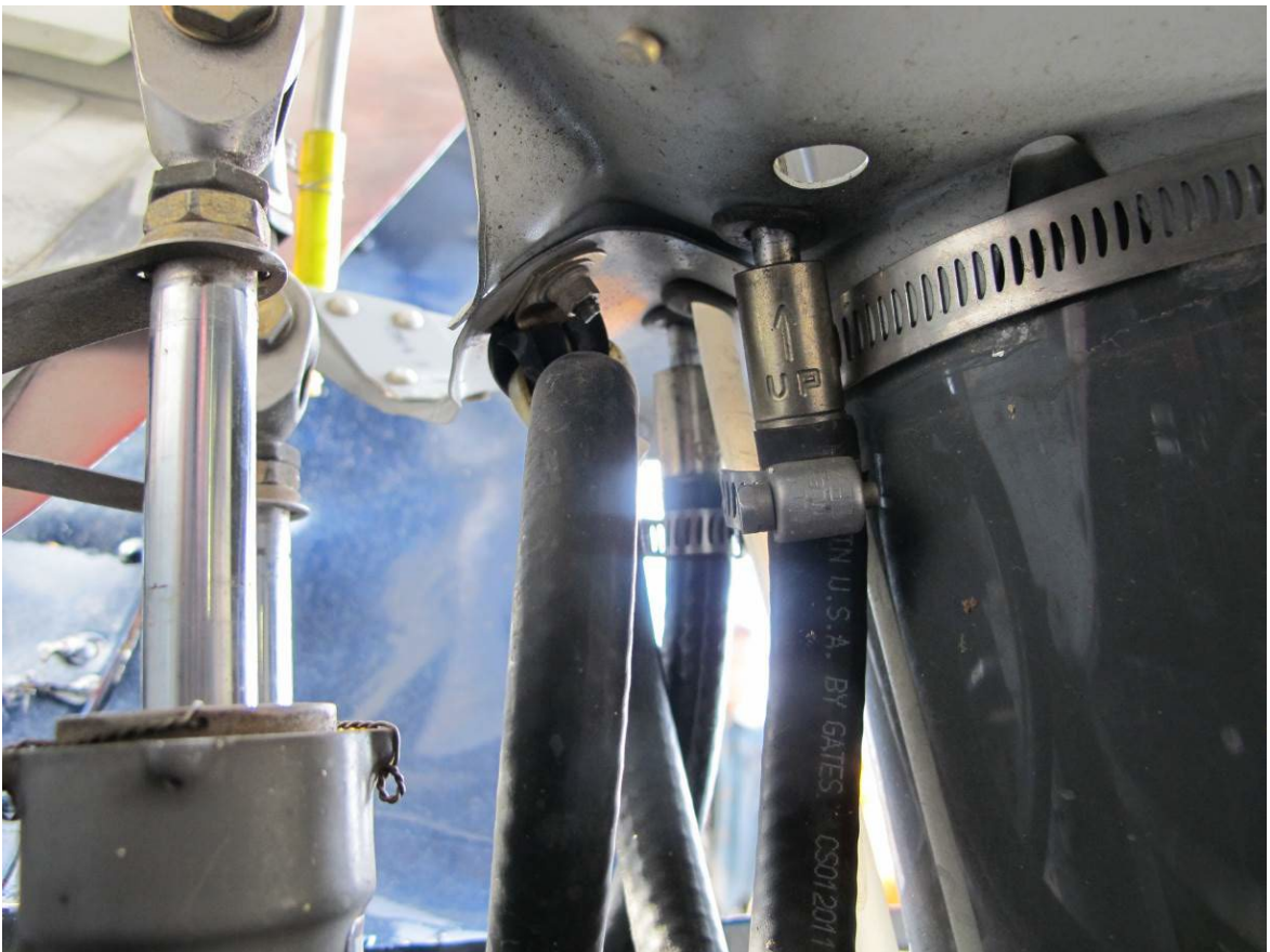
Fuel vent system rollover valves.
