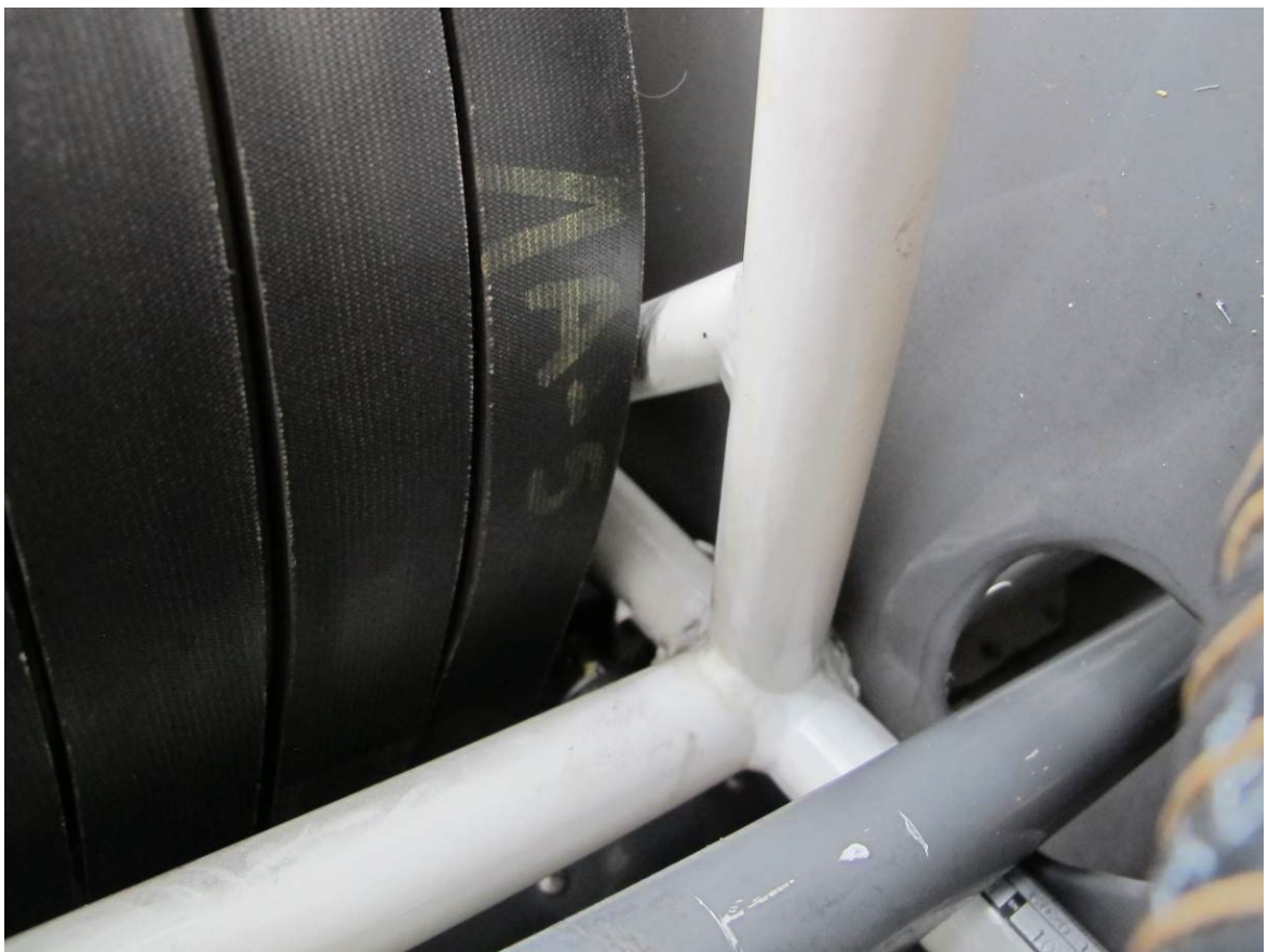
Rubber transfer on right side of upper frame.
