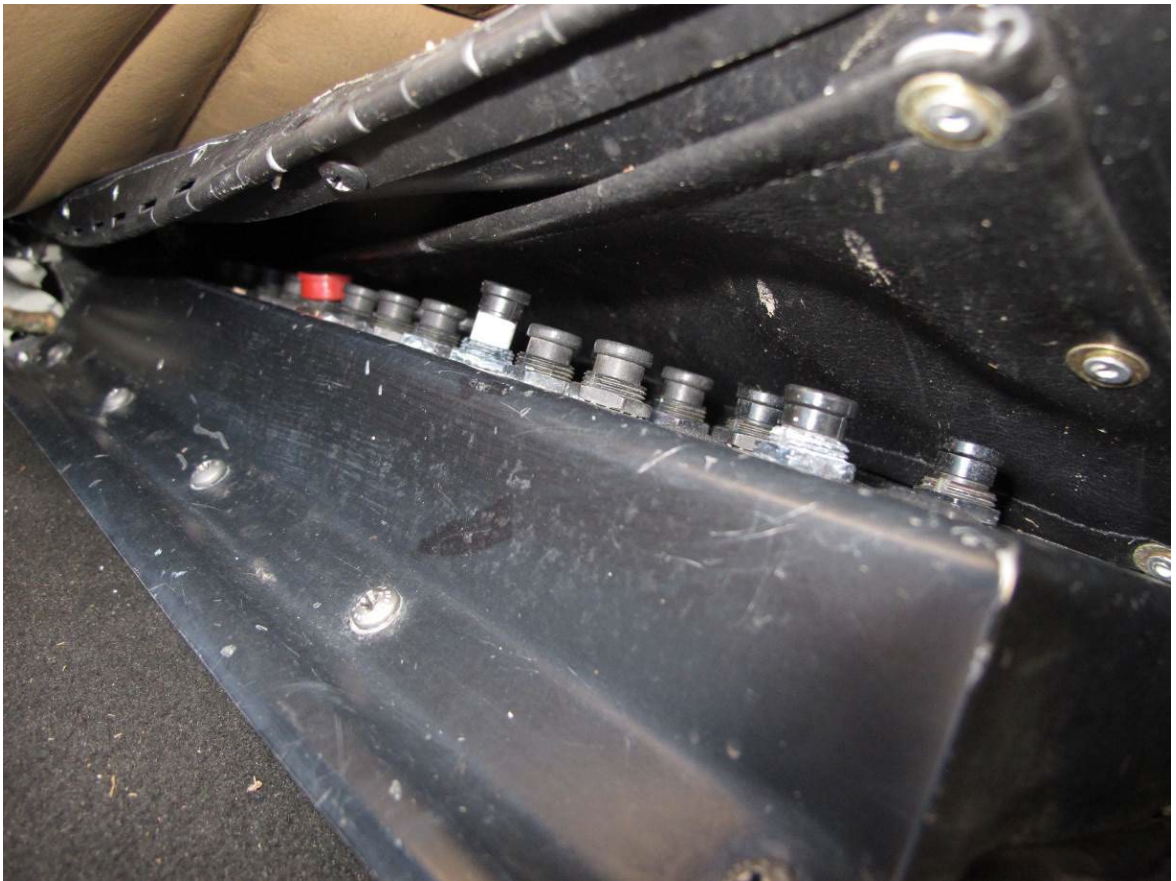
Circuit breaker panel.
