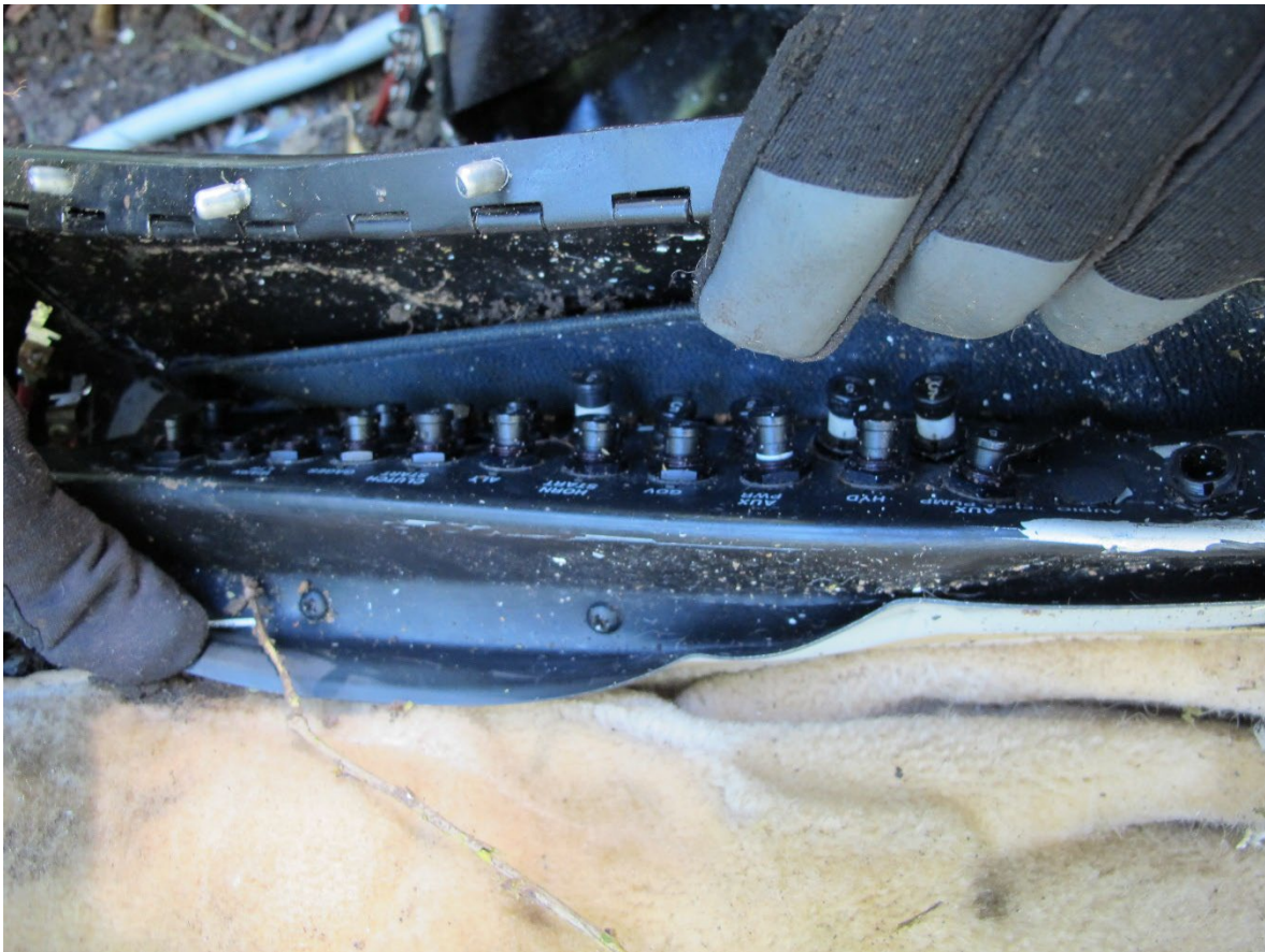
Figure 10 - Circuit Breaker Panel
