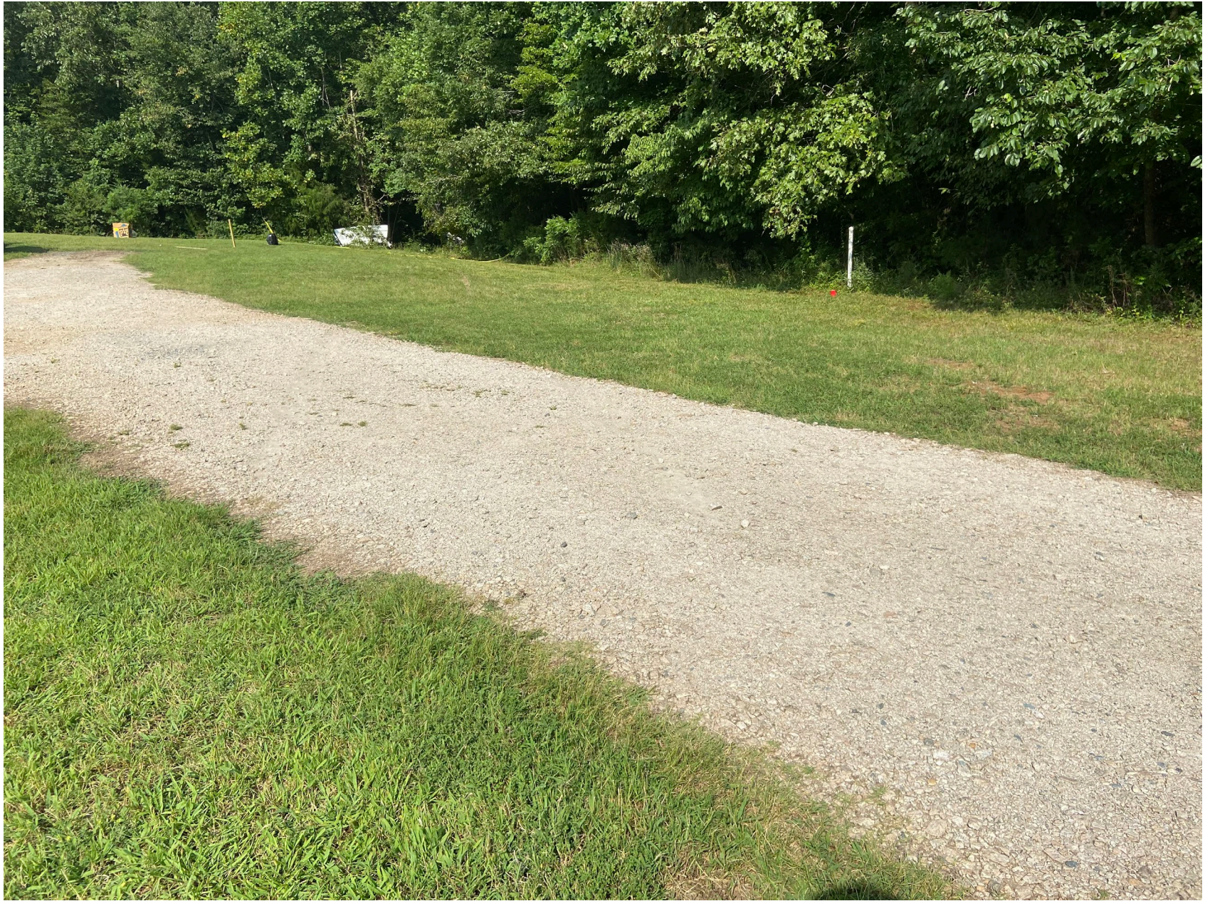
Photo 2 – Close Up of Gravel Driveway – Courtesy of FAA
