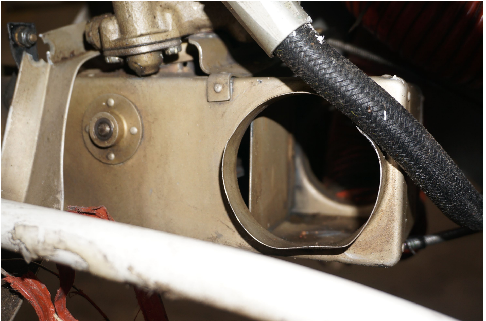
Photo 16 – Carburetor Heat Door (As Found Position)
