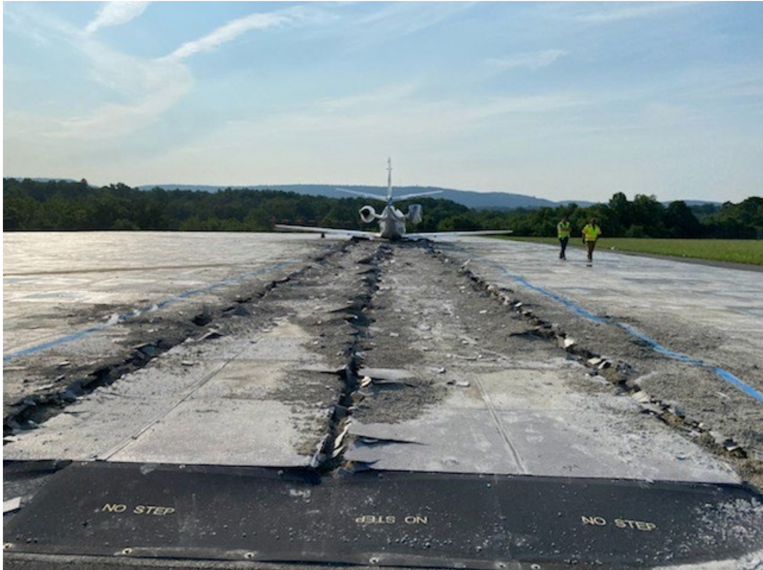
Photo 1 – View of airplane resting in EMAS system. (Courtesy of AIG)
