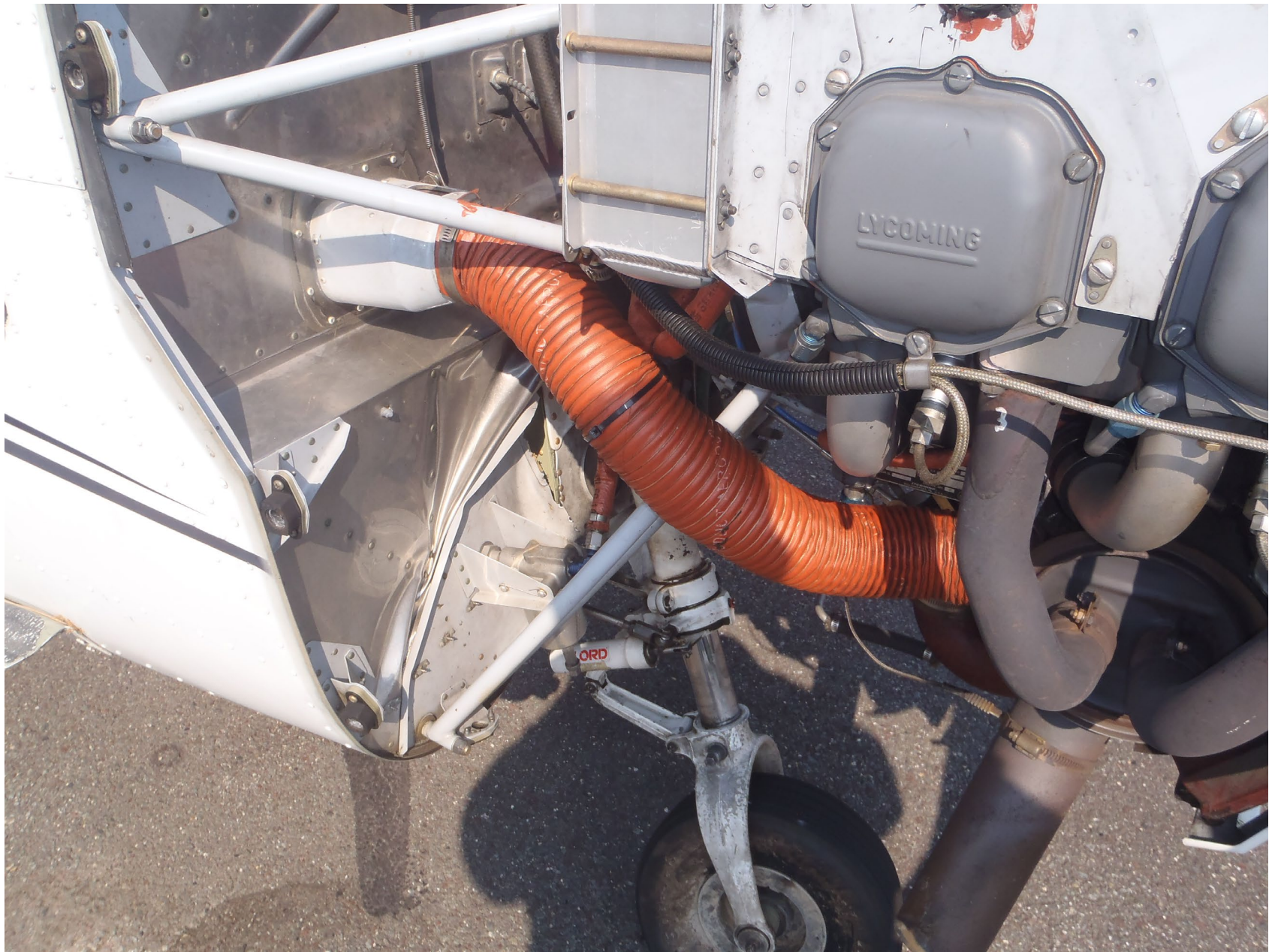
Photo 2 – View of Torn and Buckled Firewall and Nose Mount Structure (Moyer Aviation)
