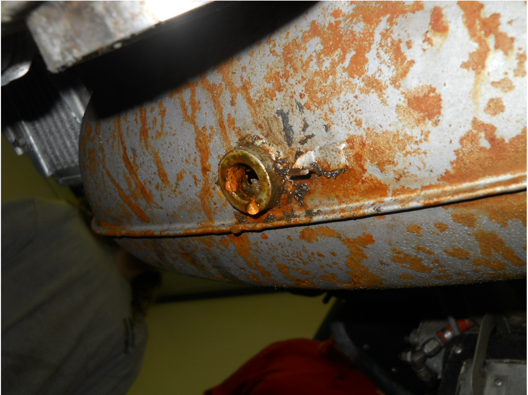
Photo 4 – Oil Sump With Missing Drain Plug
