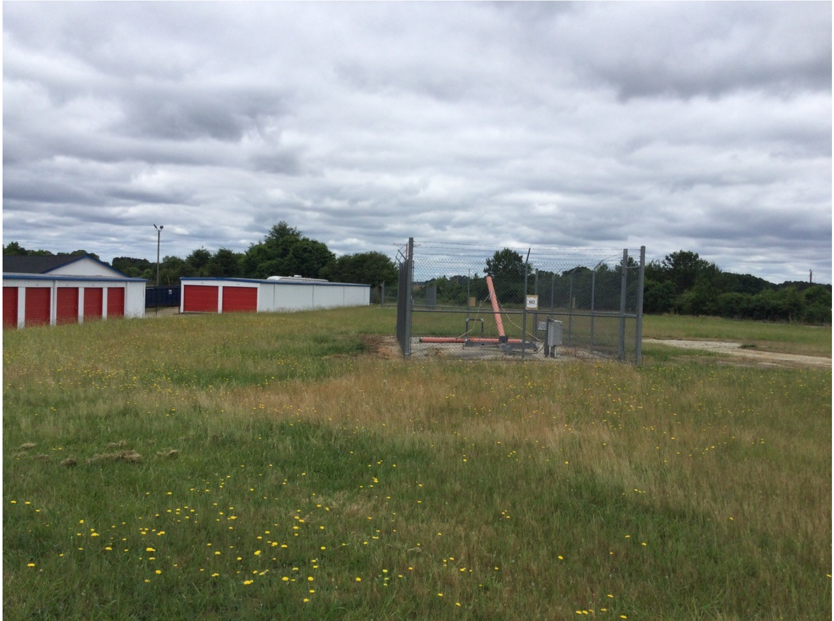
Photo 4 – View of airport approach light damage. (Courtesy of FAA)
