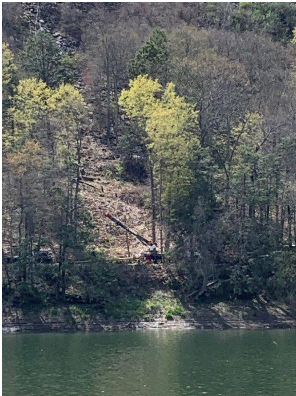
Photo 9 – View of damaged transmission pole/wires taken from opposing shore. (Courtesy of First Energy)
