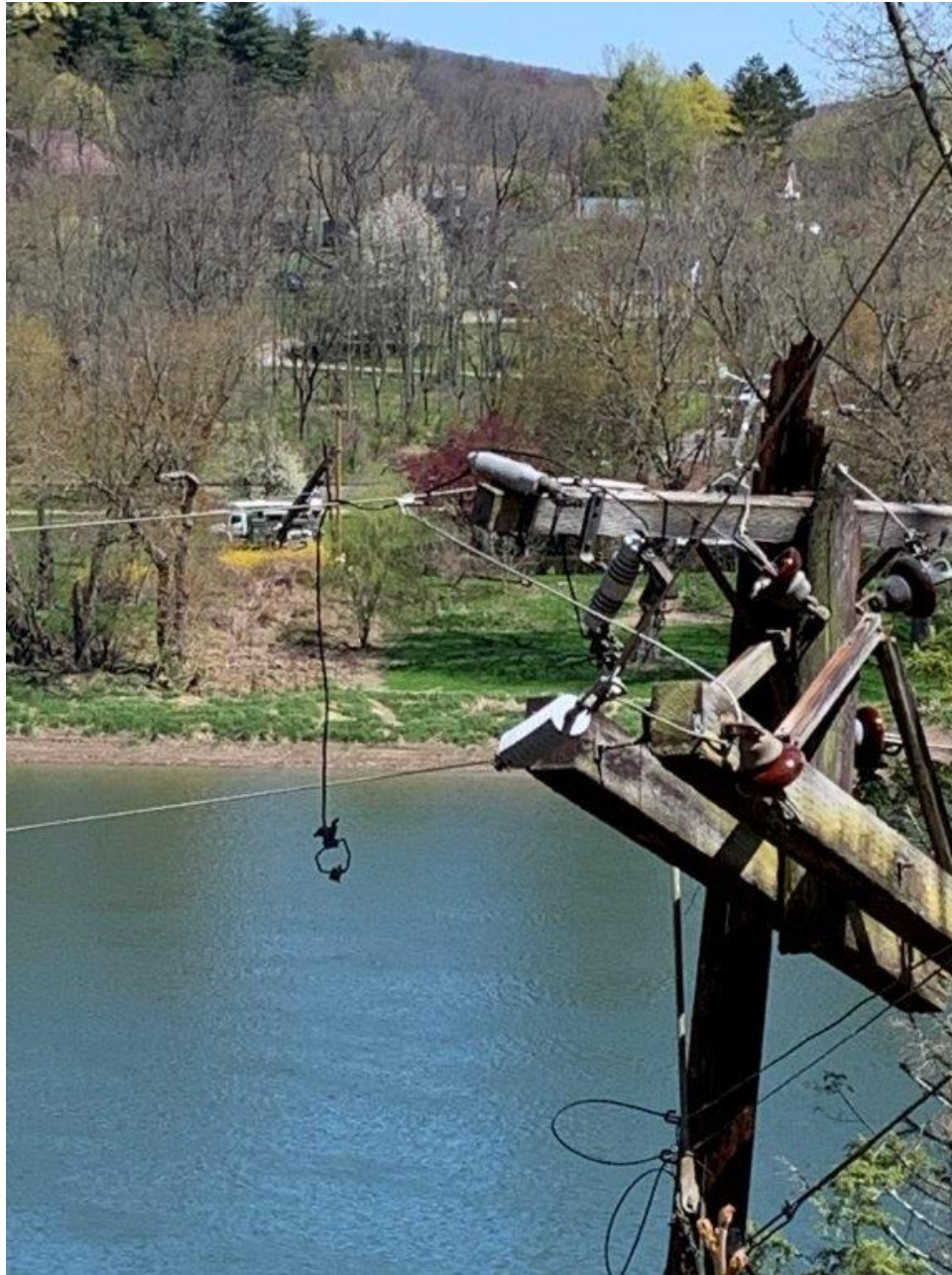
Photo 8 – Close up view of damaged transmission pole/wires. (Courtesy of First Energy)
