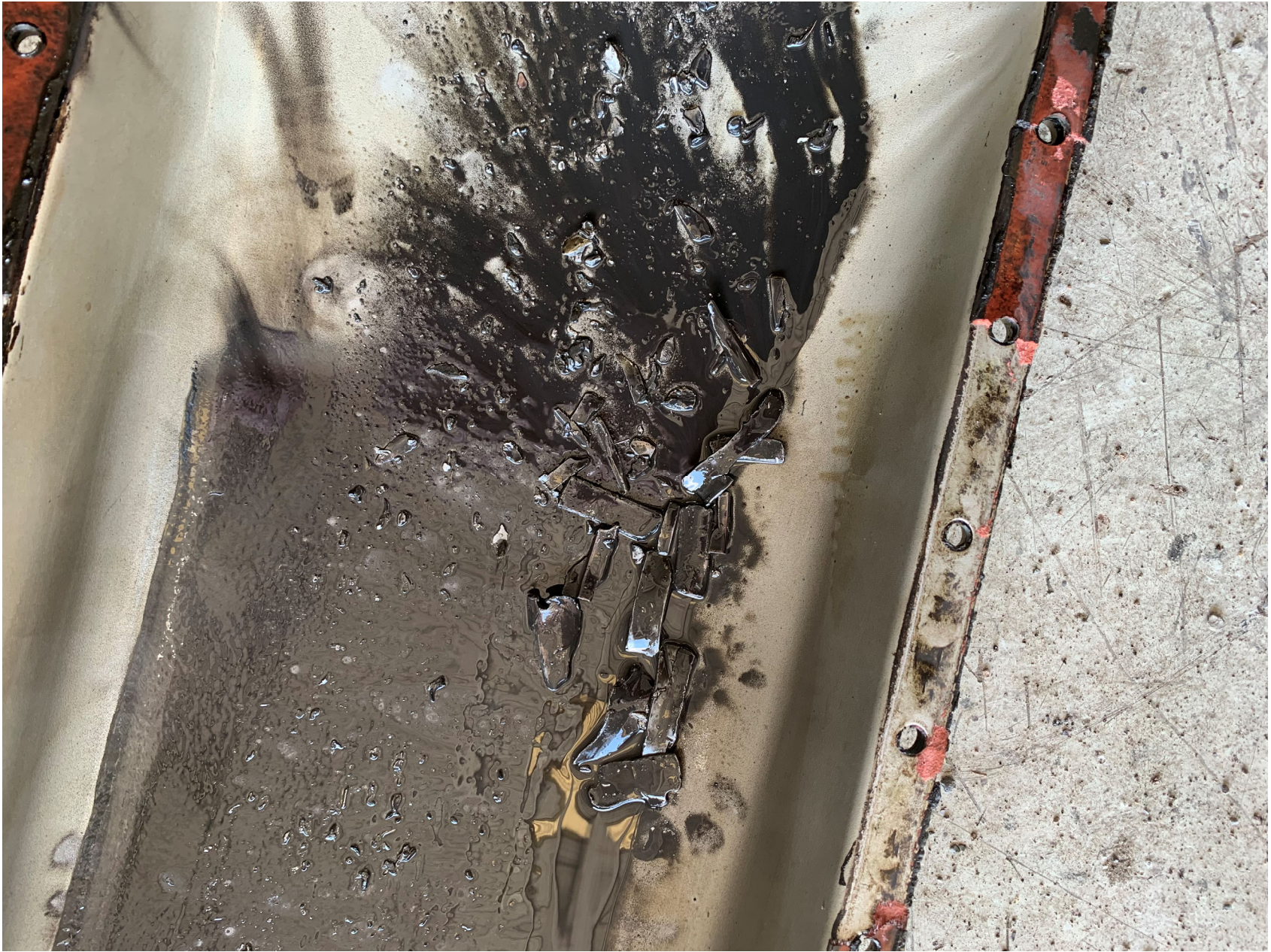
Photo 16 – Bearing Material Found in Oil Sump
