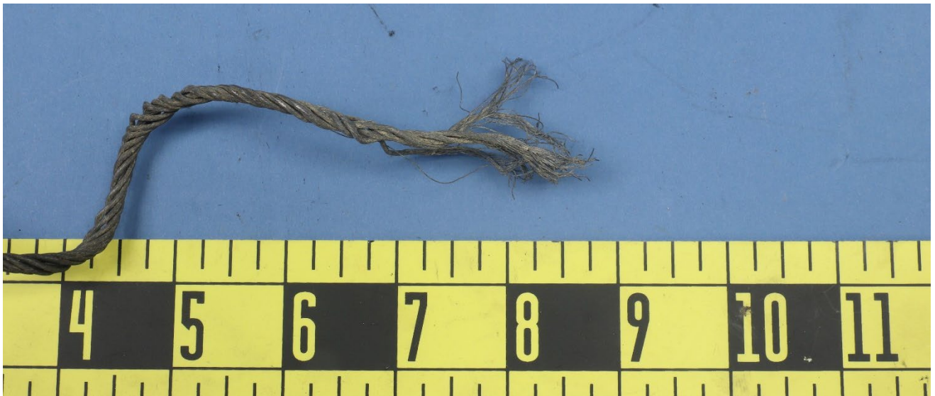
Figure 8 – View of the fractured wire strands from the opposite end, as received.
