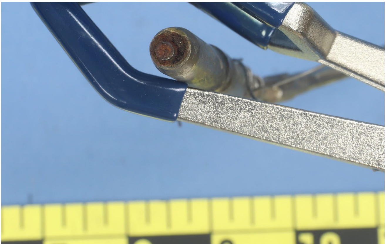
Figure 19 – View of the turnbuckle with the fractured terminal end fracture surface, as received.
