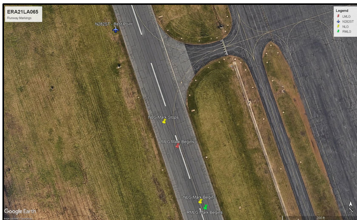
Figure 9-Rubber transfer marks on Runway 35.
