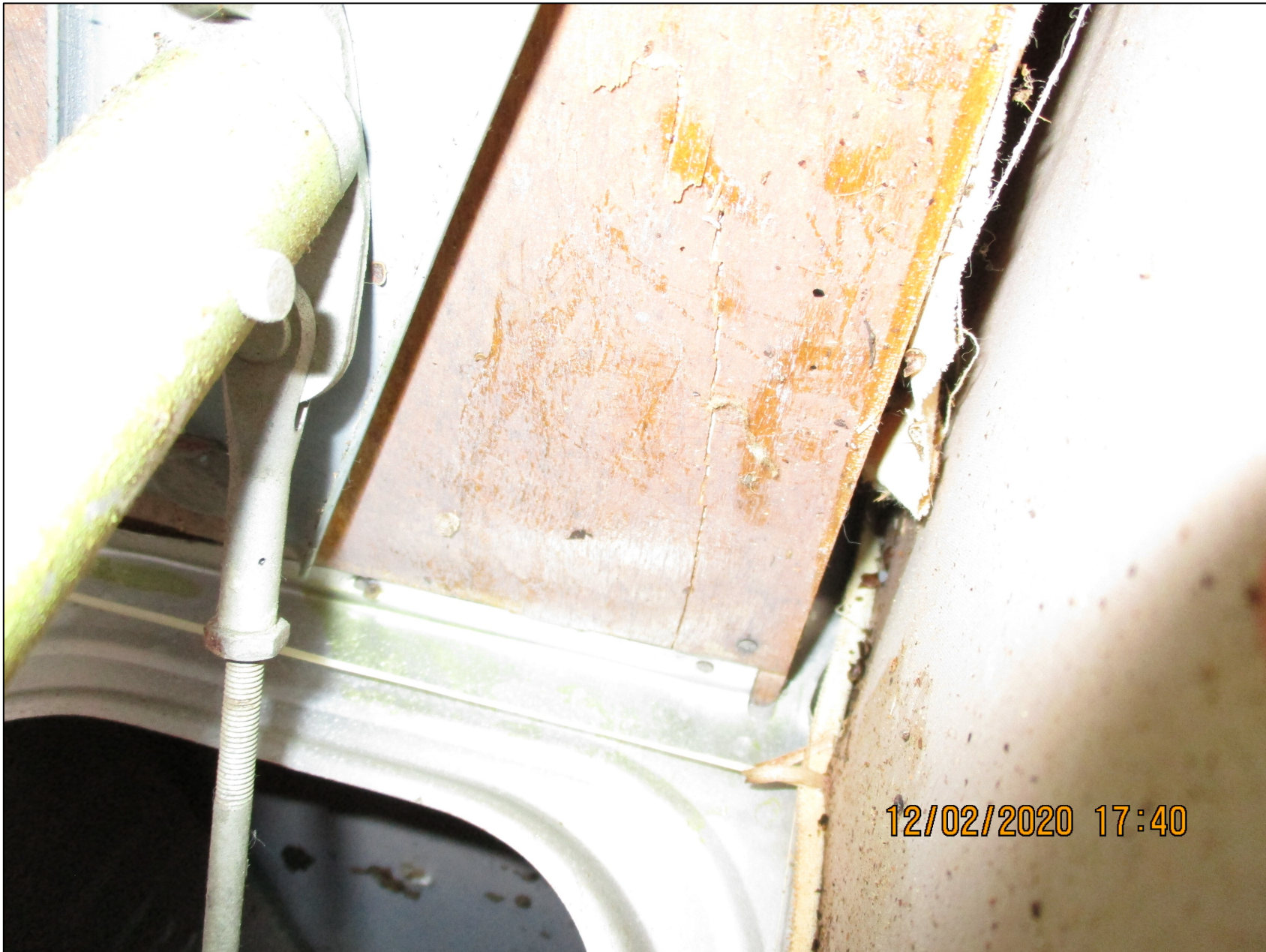
Photo 3 – View of the cracked wing spar (Photo Courtesy of FAA)
