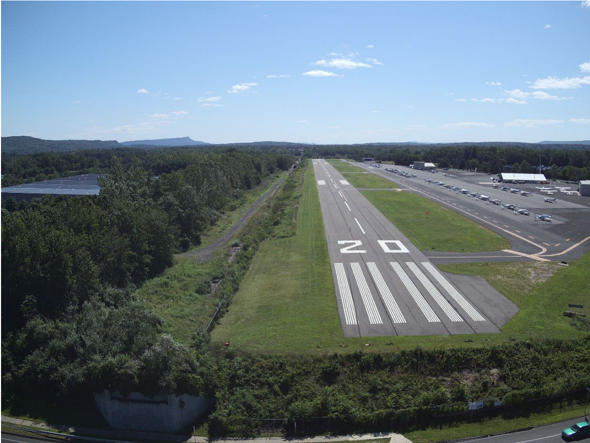
Figure 16: Still Image From UAS. View Taken Past Departure End of Runway 2 Looking Towards the Approach End of Runway 2. Note the Elevation Change Past the Departure End of the Runway.
