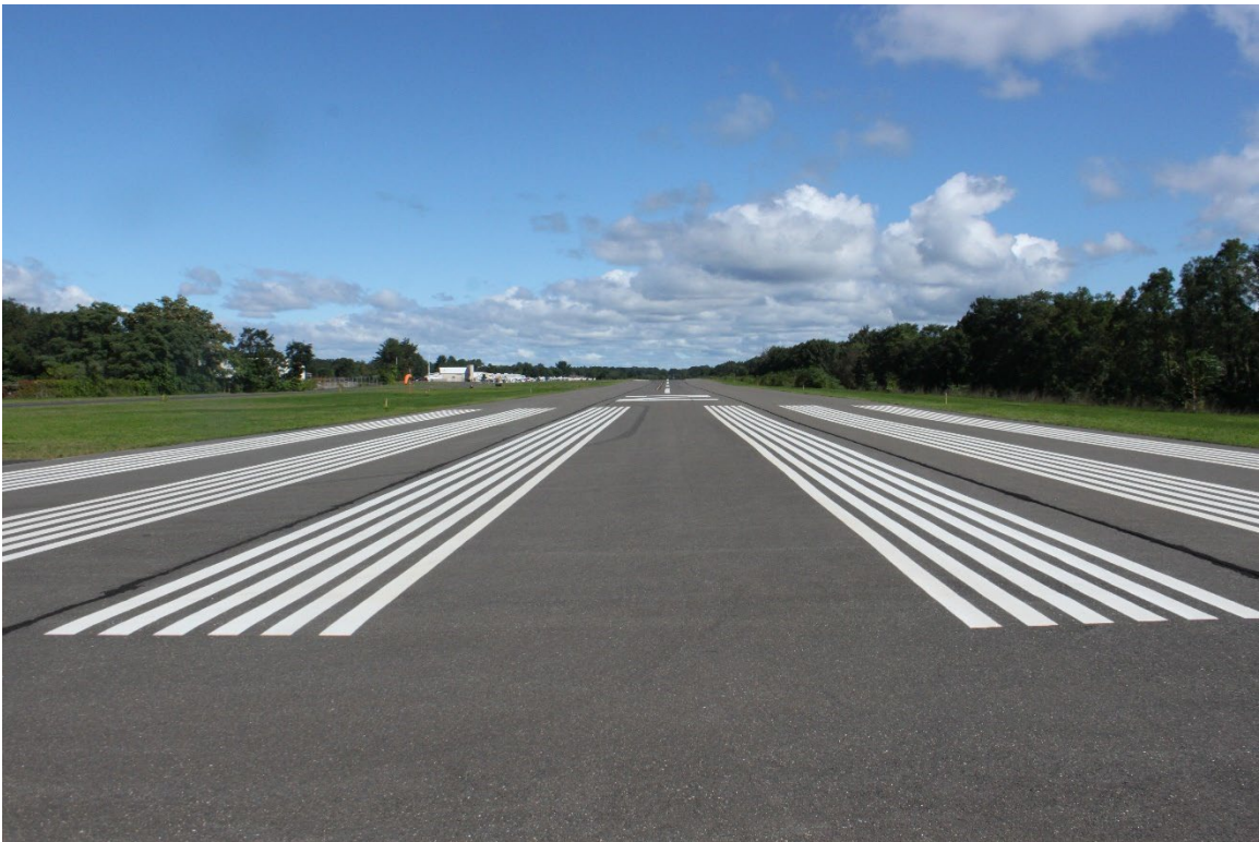
Figure 2: NTSB Digital Photograph. Ground View From Approach End of Runway 2.
