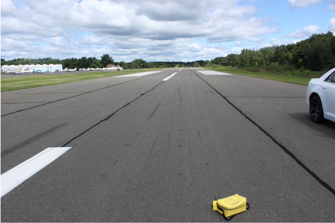
Figure 3: NTSB Digital Photograph. Yellow Bag Identifies Location of First Observed Tire Mark from Right Main Landing Gear Located 2,360.9 ft along and 9 ft right of runway centerline runway 2.
