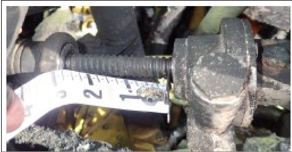
Figure 7: View of the flap jackscrew actuator
