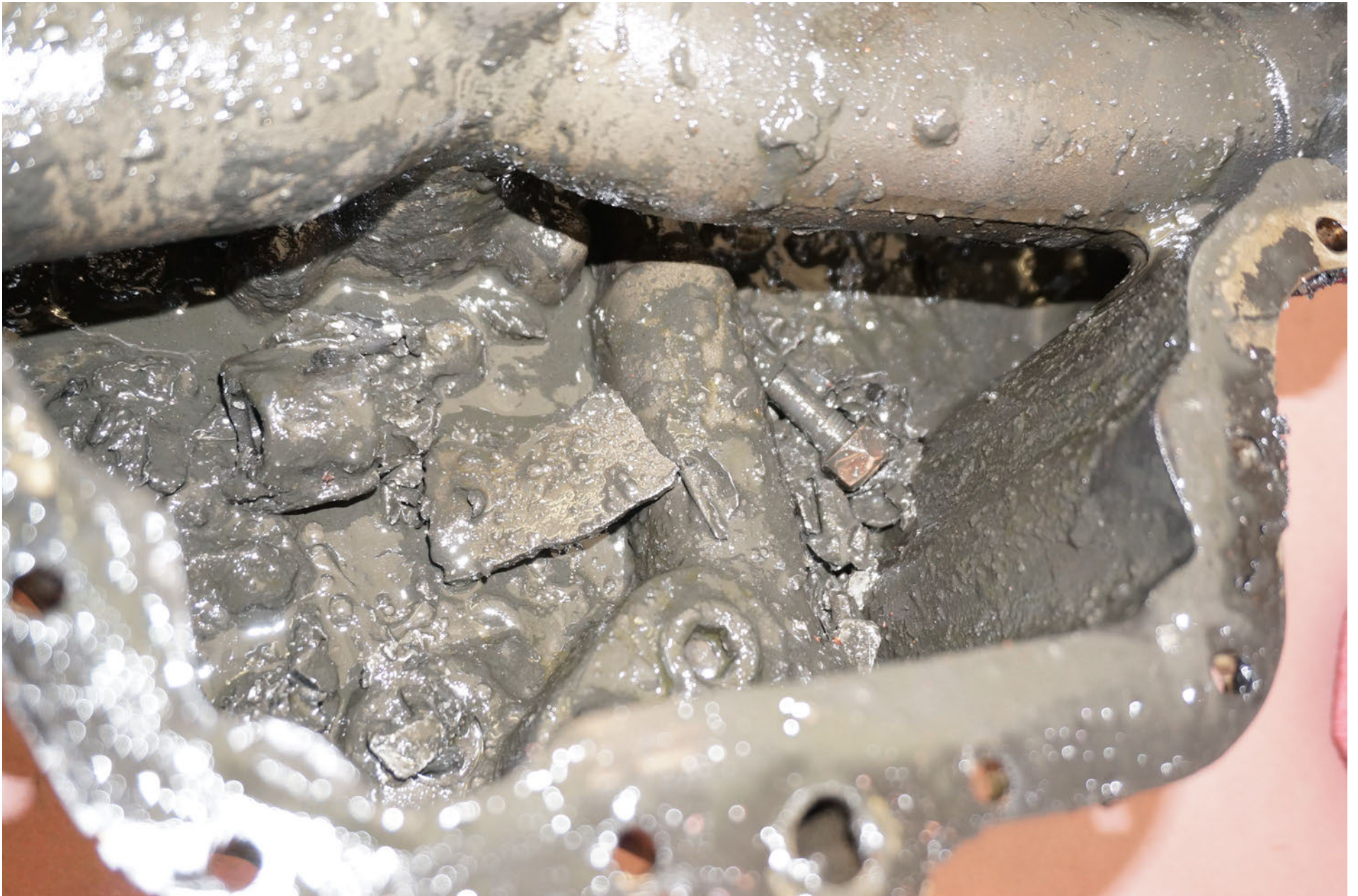
Photo 9 – Inside of Oil Sump
