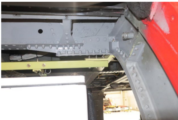
Figure 3. Water tank exterior frame right forward upper tie down attachment (typical of the top 4 corners).
