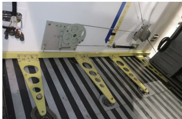
Figure 4. Water tank external frame attached to floor deck tie downs.
