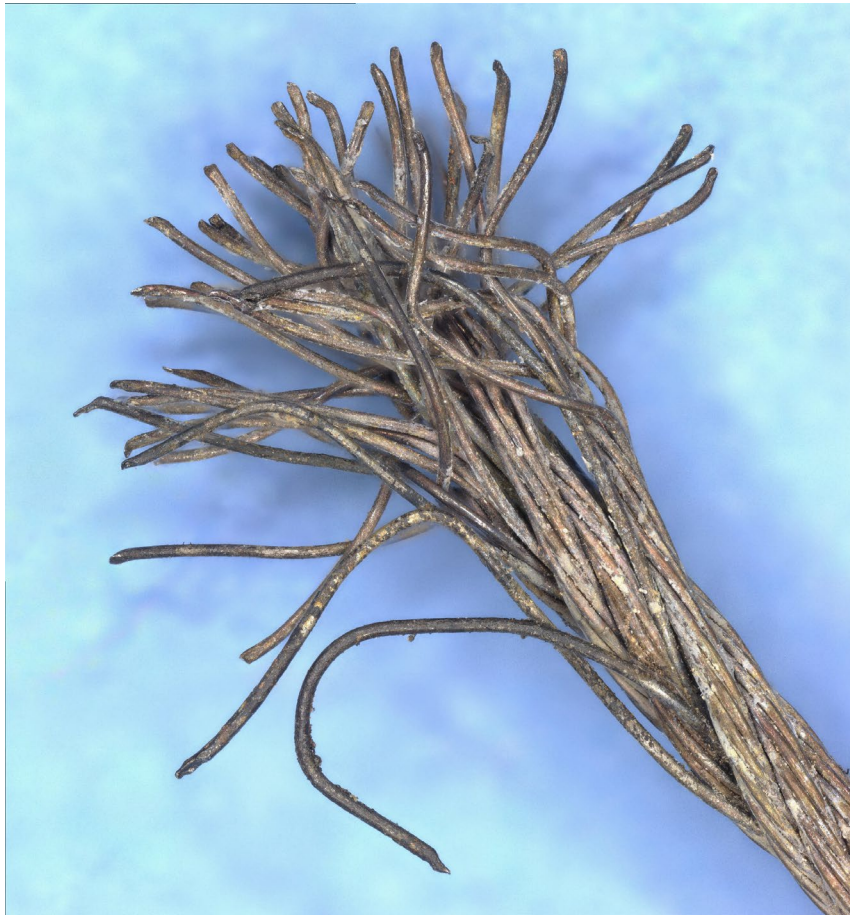
Figure 12: Cable 2/4 2-A overall view.
