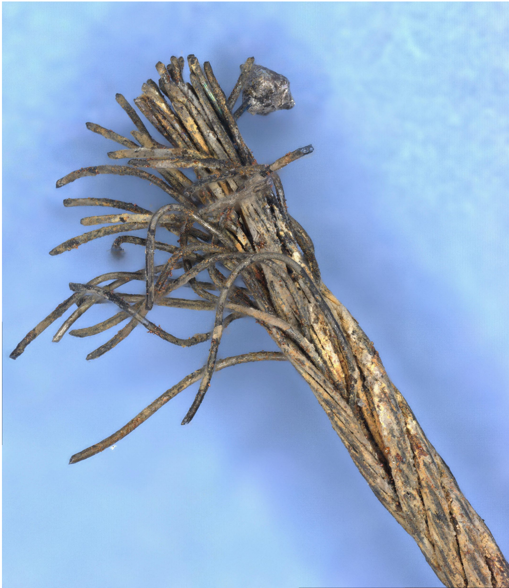
Figure 4: Cable 1/3 1-A (overall view).
