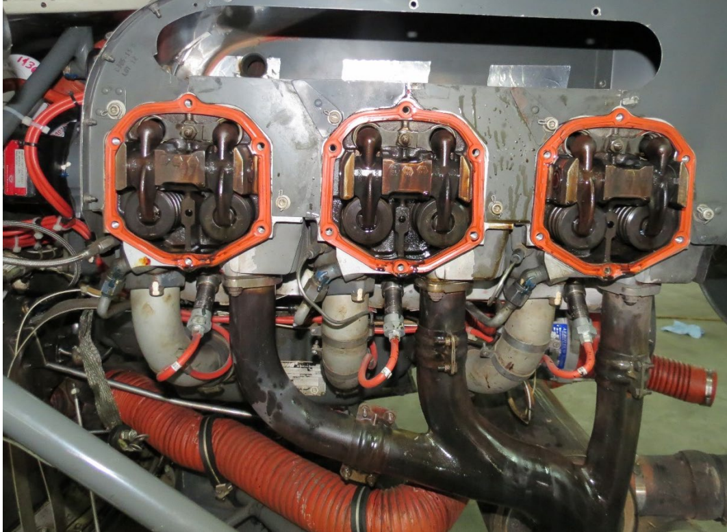
Figure 11: Engine (left) with rocker covers removed
