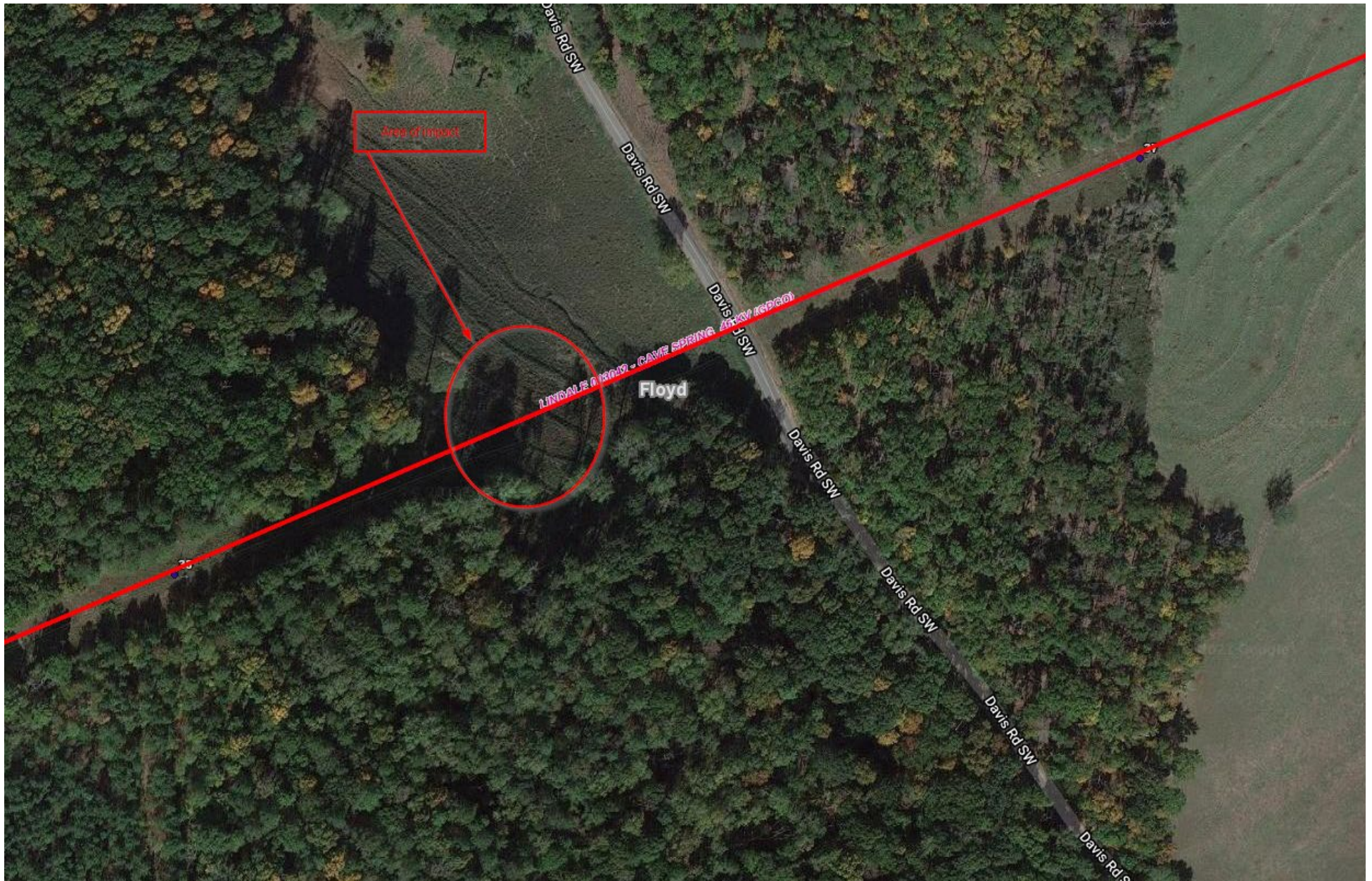
Photo 4 – Aerial view of impact point of power line. (Georgia power photo)
